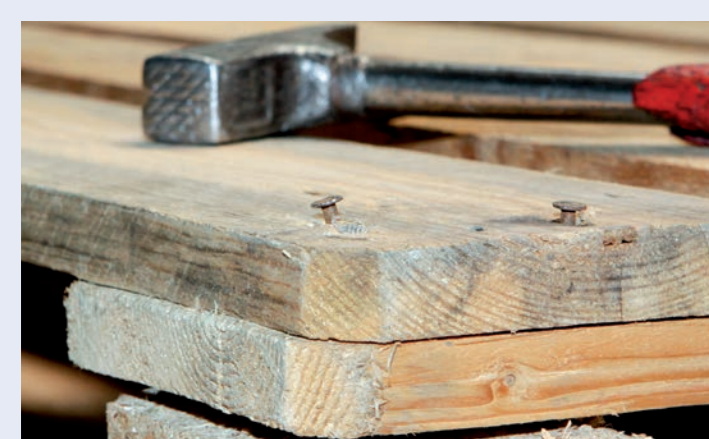
Hammering down projecting fastening elements
