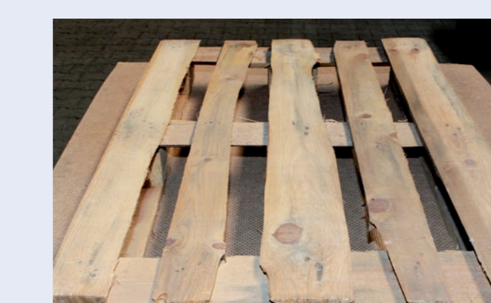
Inadmissible component e.g. underdimensioned, woodwormeaten, wane
